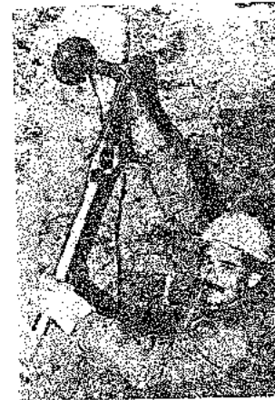
Use of a torque wrench to tension rockbolts.
