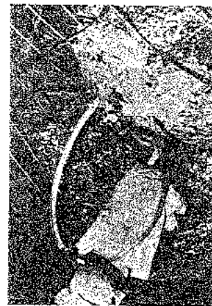
Application of rapid setting plaster to a rockbolt washer assembly to seal it for grouting.
