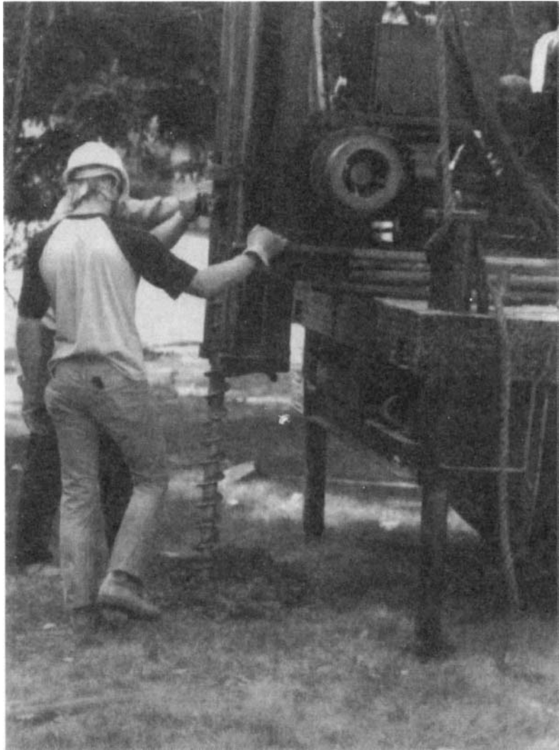
Figure 3-3 Soil drilling using a continuous-flight auger.
