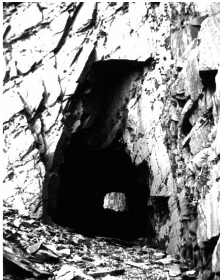
Figure 11.10: Structurally controlled failures in an old slate quarry in Wales. No support was installed in this tunnel and the final profile is defined by the wedges which have fallen from the surrounding rock mass.
