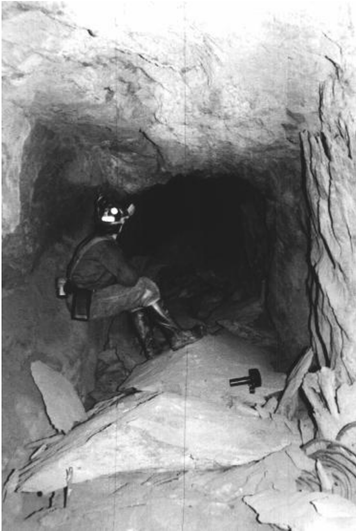
Figure 10.3: Spalling from the roof of an opening in highly stressed rock. The slabs on the floor have come from the left-hand side of the roof, just above the man's head. Spalling parallel to the right-hand sidewall is also visible.
