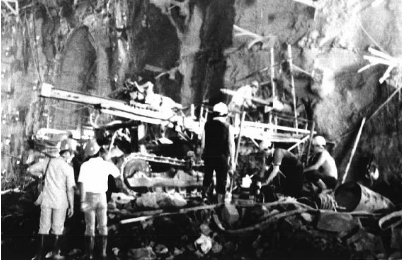
Figure 11.21: Installation of cables in the sidewall of the power cavern of the Mingtan project in Taiwan.
