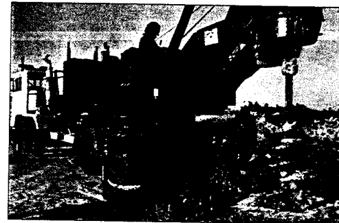
▼ Plate K Building a drilled shaft foundation ( ADSC: The International Association of Foundation Drilling )
