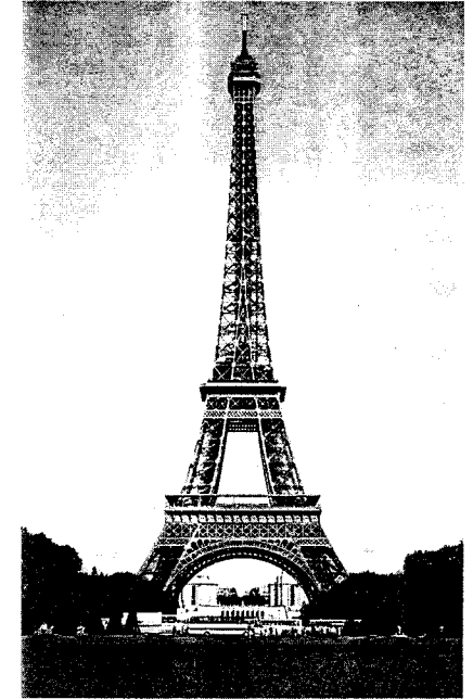
Figure 1.1 Two legs of the Eiffel Tower in Paris are underlain by softer soils, and thus could have settled more than the other two. Fortunately, Eiffel carefully explored the soil conditions, recognized this problem, and designed the foundations to accommodate these soil conditions. His foresight and diligence resulted in a well-designed foundation system that has not settled excessively.
