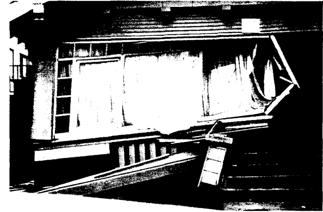
Figure 9.30 House that separated from its foundation during the 1989 Loma Prieta Earthquake (Photo by C. Stover, U.S. Geological Survey).
