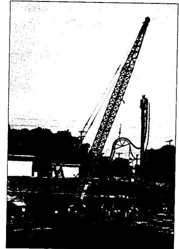
▶ Plate L Using a vibrofloat to install a stone column
