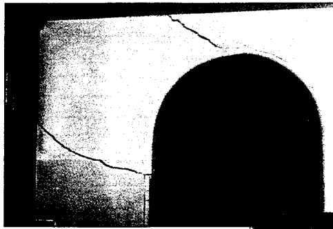
◀ Plate E Cracks in the interior walls of a house that experienced excessive differential settlements
