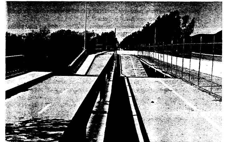
Figure 8.21 Deck view of the bridge shown in Figure 8.20. The lanes on the right side of the fence are supported by a separate pier that was not undermined by the scour.
