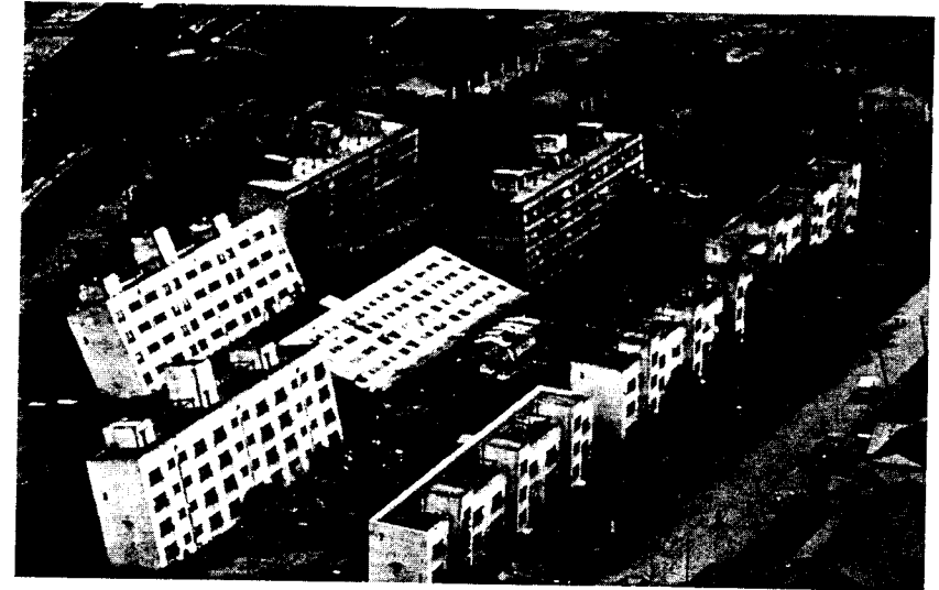
Figure 8.9 The soils beneath these apartment buildings in Niigata, Japan liquefied during the 1964 earthquake, which produced bearing capacity failures. These failures reportedly occurred very slowly, and the buildings were very strong and rigid, so they remained virtually intact as they tilted. Afterwards, the occupants of the center building were able to evacuate by walking down the exterior wall (Earthquake Engineering Research Center Library, University of California, Berkeley, Steinbrugge Collection).
