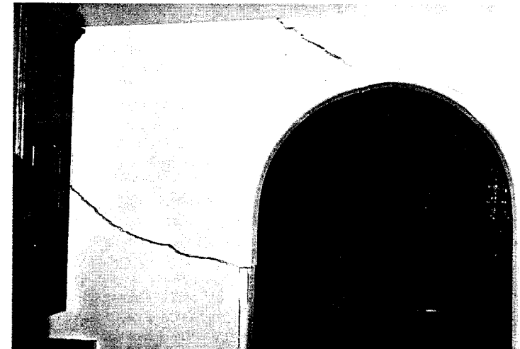
Figure 2.6 This wood-frame house was built on an improperly compacted fill, and thus experienced excessive differential settlements. The resulting distortions produced drywall cracks up to 15-mm wide, as shown in this photograph, along with additional cracks in the exterior walls and the floor slab.
