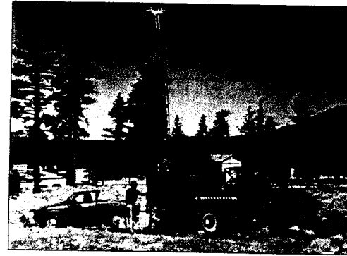
◀ Plate I Drilling an exploratory boring
