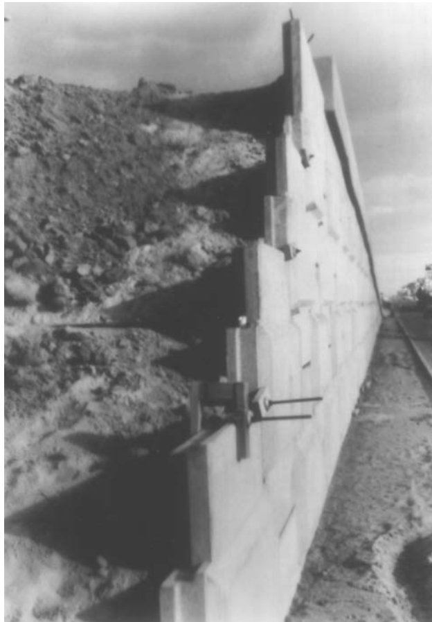
Figure 8.26 Reinforced-earth retaining wall (with metallic strip) under construction (Courtesy of Braja M. Das, Henderson, NV)
