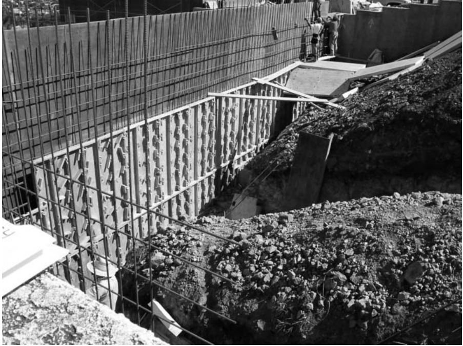
Figure 8.2 A cantilever retaining wall under construction (Courtesy of Dharma Shakya, Geotechnical Solutions, Inc., Irvine, California)
