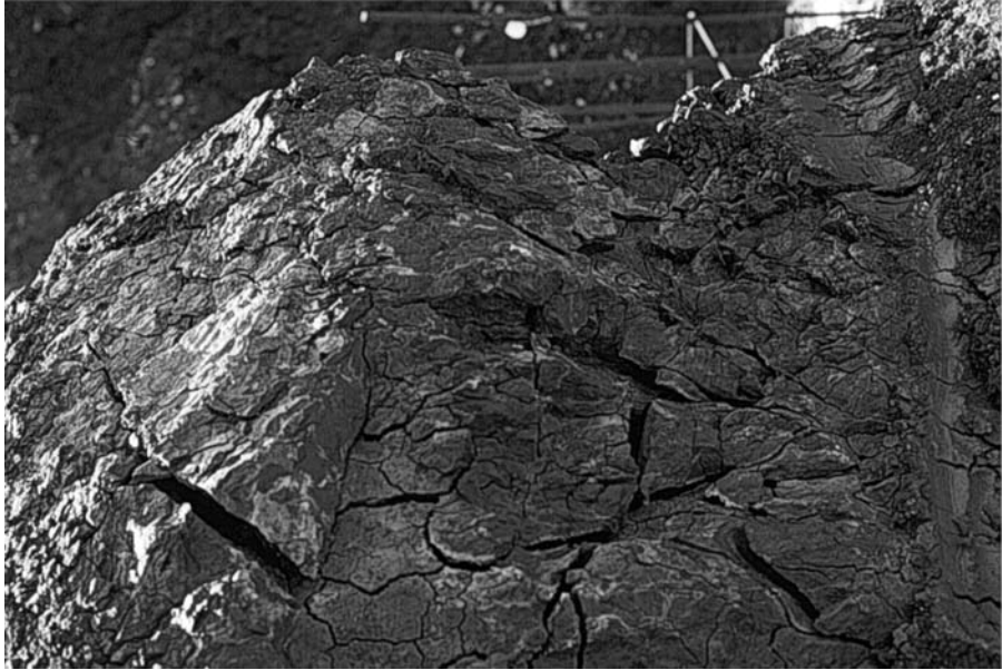
Figure 13.12 Interconnected shrinkage cracks extended from the ground surface into the active zone (Courtesy of Thomas M. Petry, Missouri University of Science and Technology, Rolla, Missouri)
