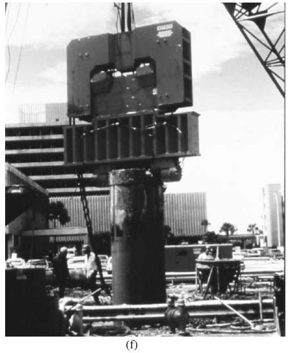
Figure 11.7 (continued) Pile-driving equipment: (c) double-acting and differential air or steam hammer; (d) diesel hammer; (e) vibratory pile driver; (f) photograph of a vibratory pile driver (Courtesy of Michael W. O'Neill, University of Houston)
