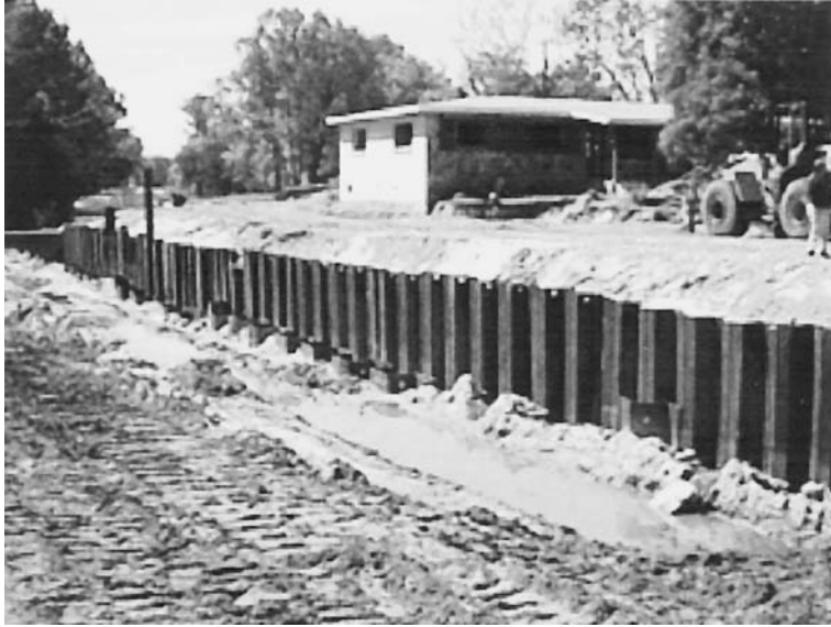
FIGURE 15.1 A flexible retaining wall under construction.
