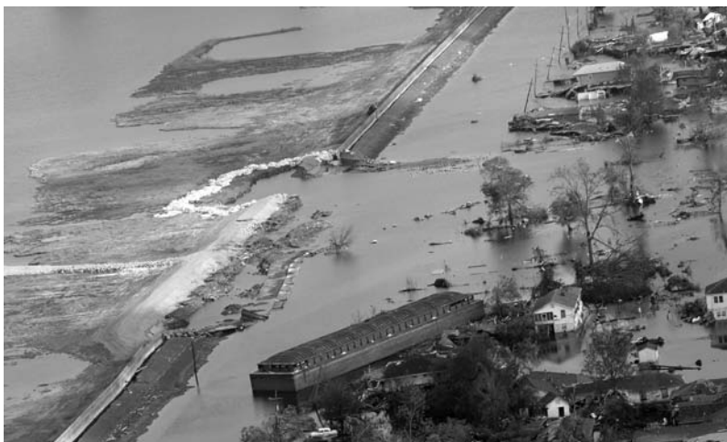
FIGURE 5.1 Failure of a section of a levee from Hurricane Katrina. (© ROBYN BECK/AFP/Getty Images/NewsCom.)
