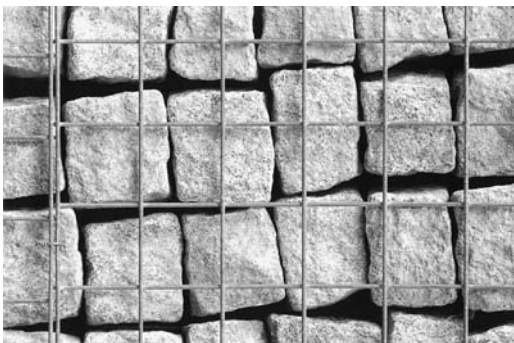
FIGURE 15.32 Gabion basket wall. (Alamy Images.)
