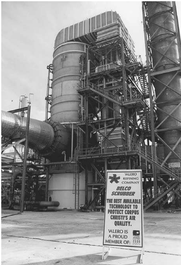
FIGURE 11.2.1 EDV wet scrubbing system in Texas.
