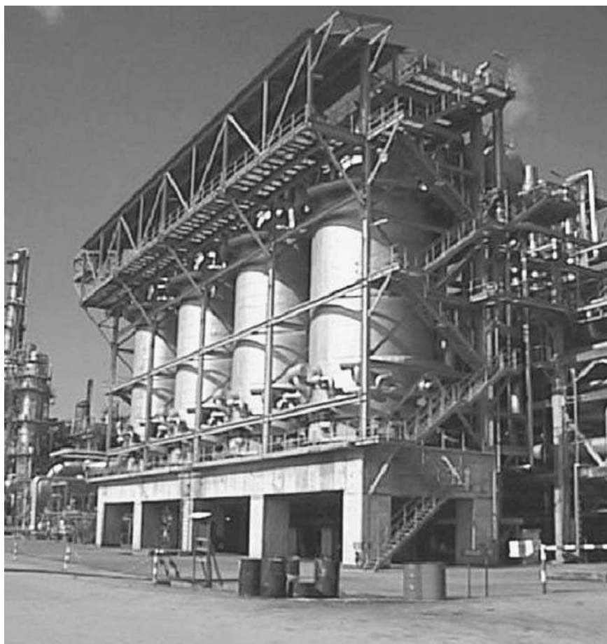
FIGURE 15.3.7 Fixed-bed multitubular (FT) reactors of SMDS Bintulu, Malaysia.
